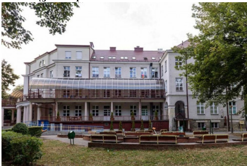
The "Górka" Specialist Chiropractical-Rehabilitation Hospital
