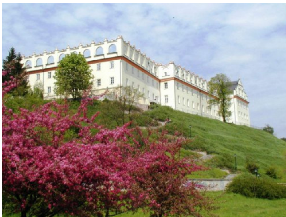
Collegium Gostomianum. The architectural shape of the site has remained unchanged
