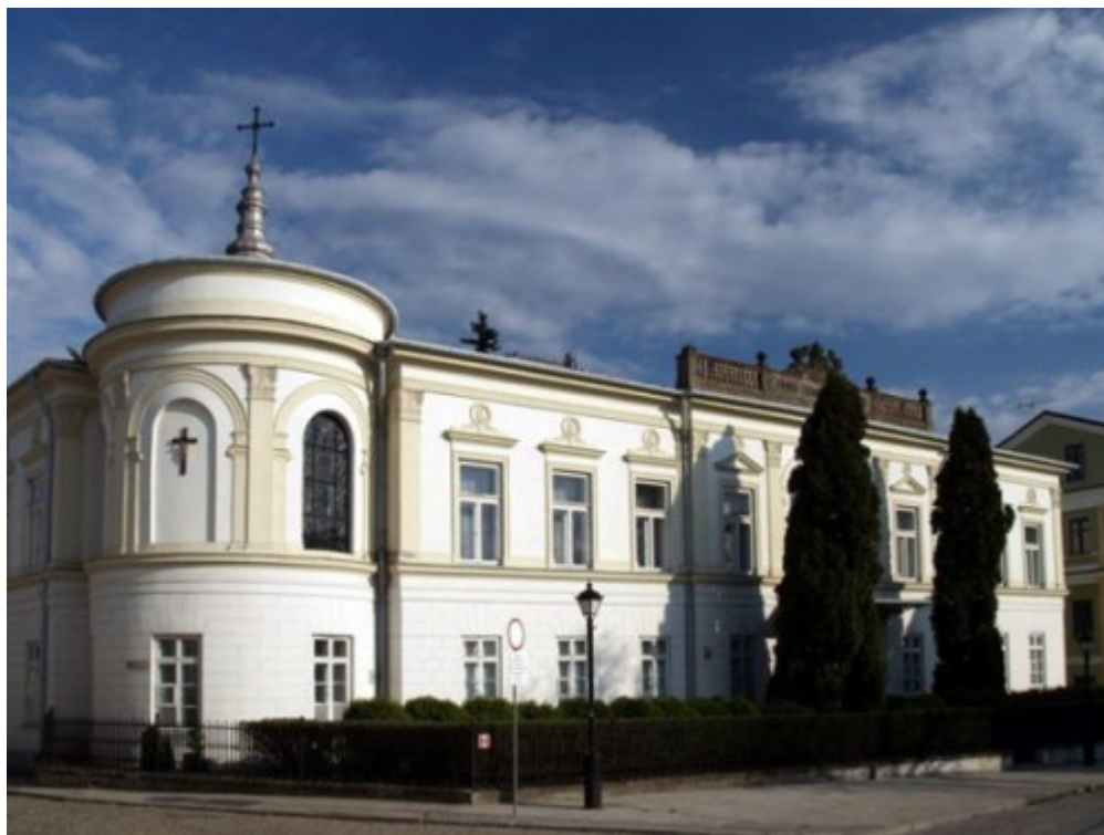
A classical building with a low attic
